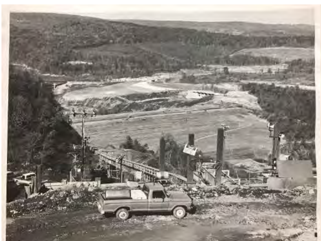
Jennings Randolph Lake (Bloomington Dam) under construction
