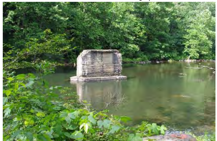
Former vehicular bridge pier
