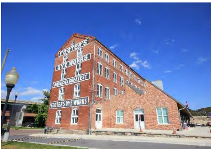
Footer Building (1906) Adaptive Reuse project
