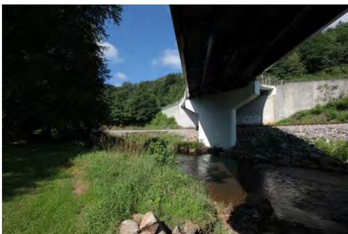
The railroad passes underneath US Route 50 on the Maryland side of the North Branch.
