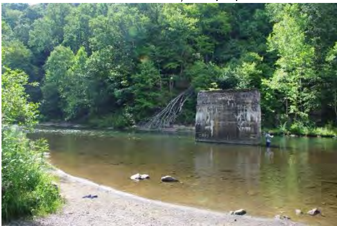
Former coal tram/conveyor pier
