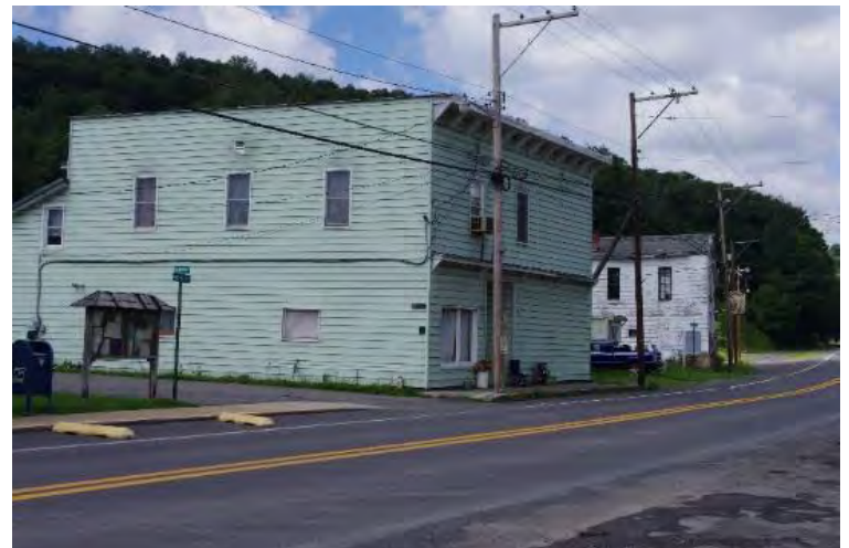
Commercial buildings across from railroad
