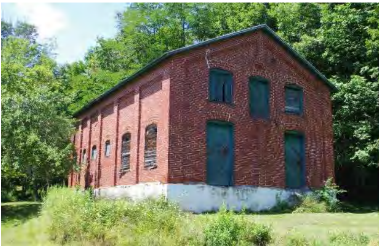
Buxton & Landstreet Company Store Warehouse. Because company stores were illegal in Maryland, the Kempton store was built across the state line in West Virginia
